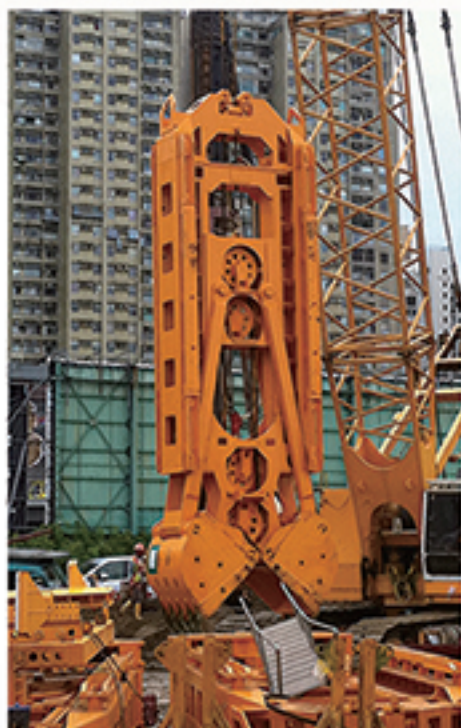
Diaphragm wall cutting
