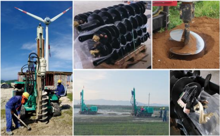
Auger (Soil Precast piles)
