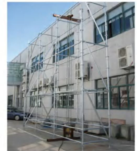
Ringlock Tower (One unit test)
