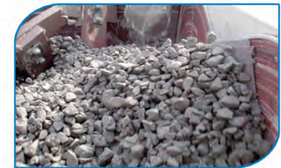
Test running with 10% overloaded dry aggregate
