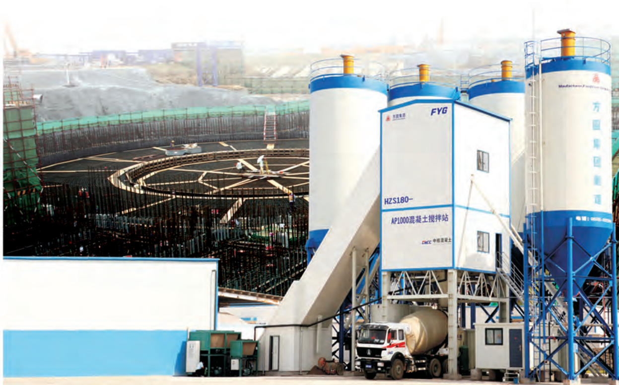
▲ Precooling concrete mixing for nuclear island construction
