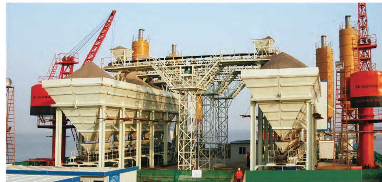
▲ Mixing plant on water platform
