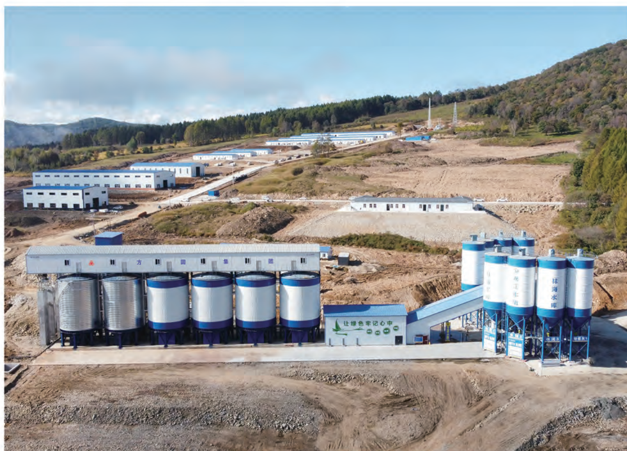
▲ Aggregate-precooling concrete mixing for dam construction
