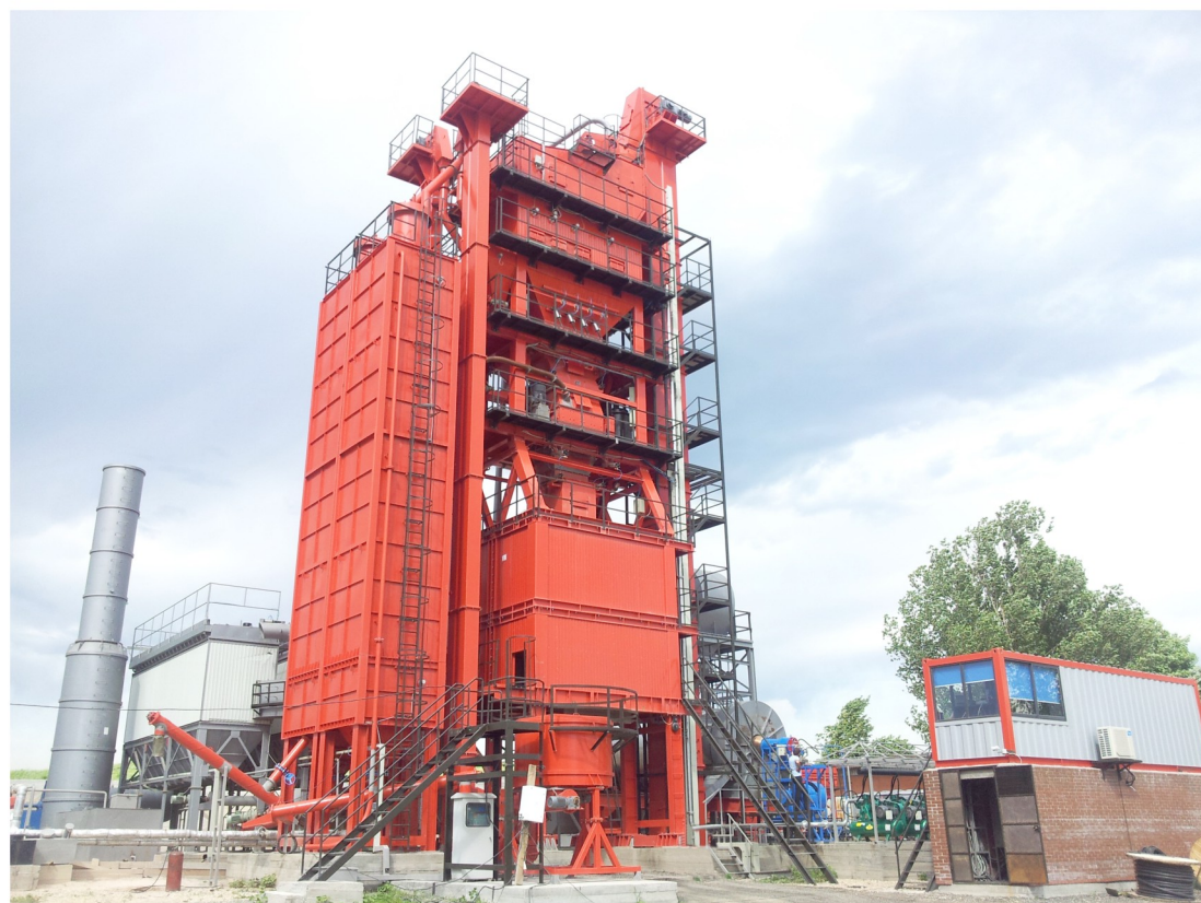
AMP2000-C (storage silo underside)
