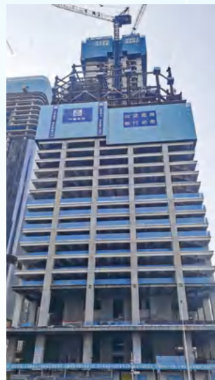
深圳科技联合大厦 Shenzhen Science And Technology Union Building
