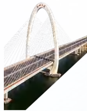
韶州大桥 Shaozhou Bridge 110m
