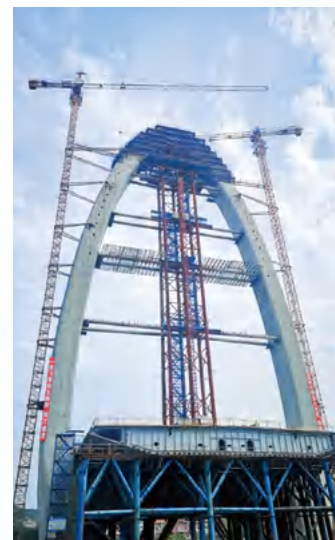
韶州大桥 Shaozhou Bridge
