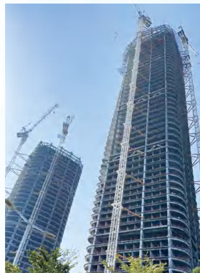
珠海横琴总部大厦 Hengqin Headquarters Building, Zhuhai
