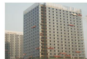
Shopping mall construction
