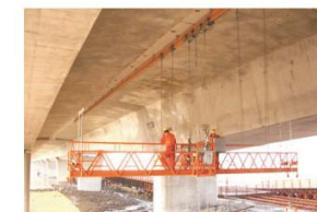
Bridge floor construction
