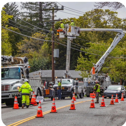
Power & Telecommunications Maintenance
