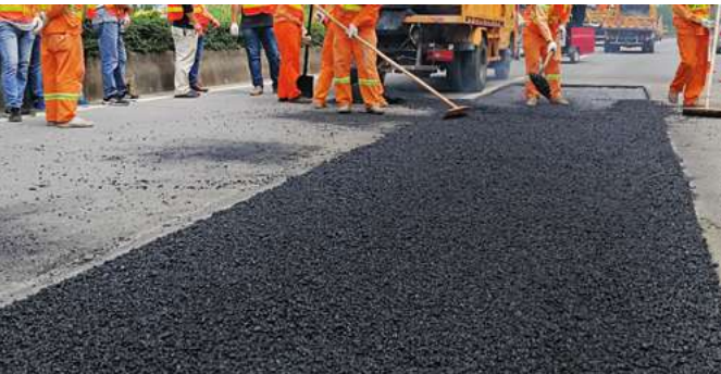
On-site transportation and paving
