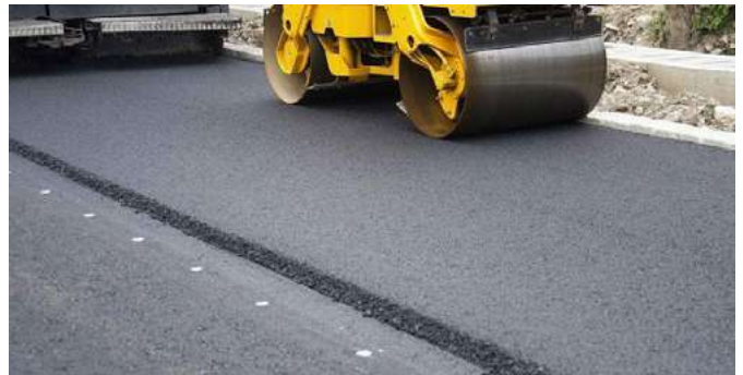
Realization of reclaimed asphalt utilization
