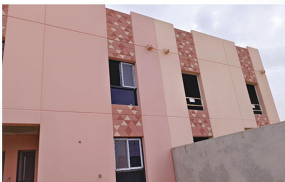
混凝土装配式建筑 Concrete prefabricated building
