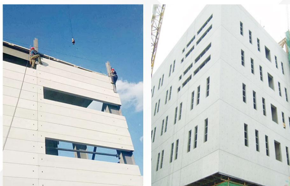
钢结构 / 混凝土结构外挂板 External wall panels for steel/concrete structures
