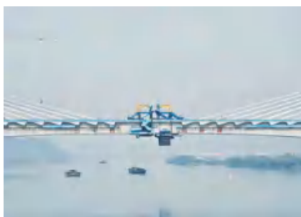
Changtai Yangtze River Bridge 常泰长江大桥
