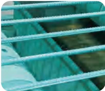
Rebar in Epoxy surface 环氧表面钢筋
