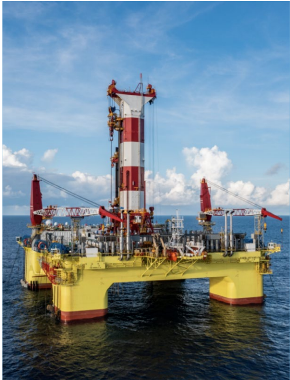
钻井平台 Drilling platform
