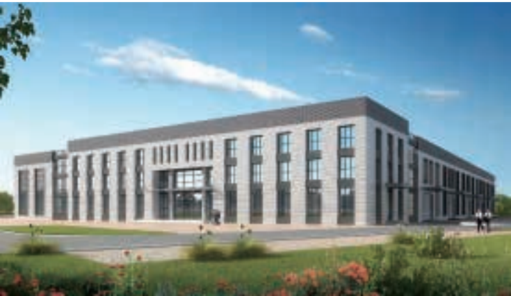
华全电力研发中心 Huaquan Electric Power R&D Center
