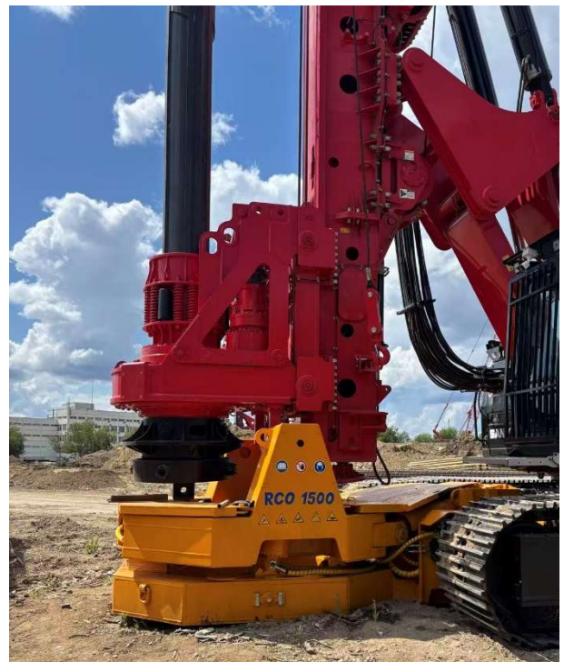
RCO 1500 with SANY Drilling rig
