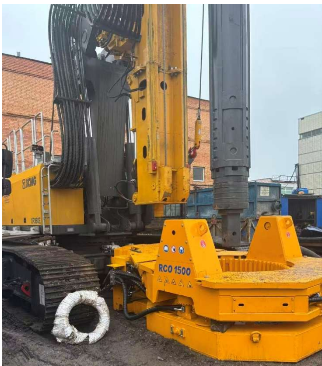
RCO 1500 with XCMG Drilling rig
