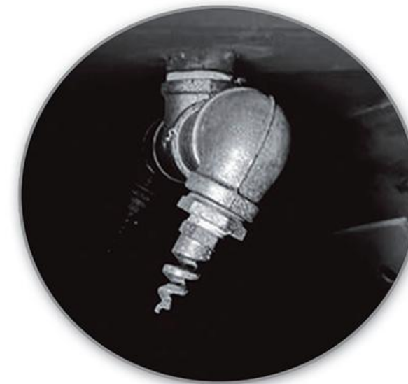
The water supply system employs both overhead and integrated piping, effectively eliminating residual admixtures and water retention in the lines
