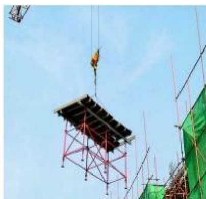
钢支撑在台模中的应用 Application in tableform formwork
