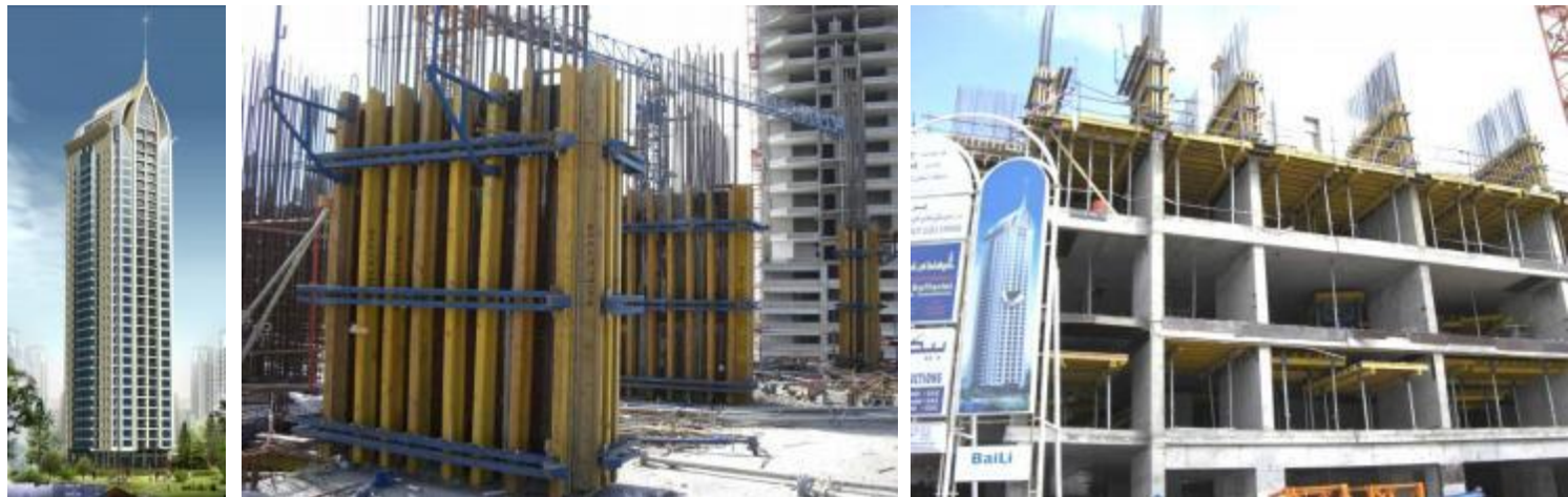
© Project located in Ajman, U.A.E
