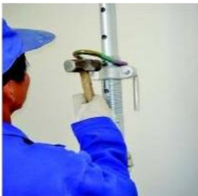
(8) 钢销退出后，回缩内管 Retrieval of inner tube after the removal of bolt
