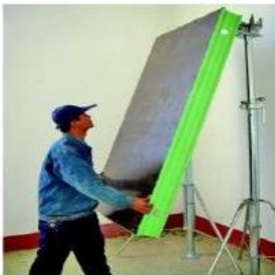
(5) 采用独立钢支撑进行顶板模板的支设 Support the slab panel with steel props
