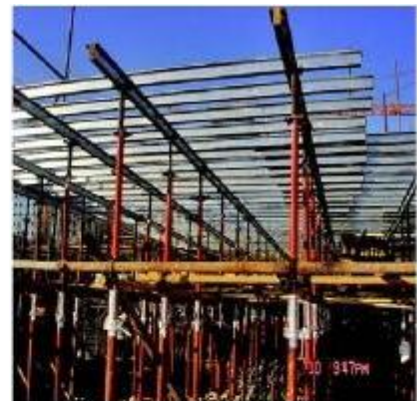
(6) 采用几字梁等材料进行顶板模板的支设 Support the slab formwork with steel & wood beam
