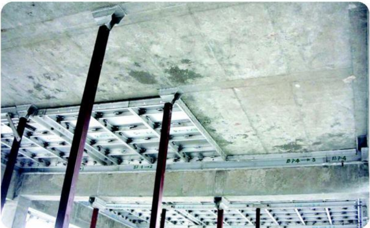
拆除模板 Dismantle the Formwork
