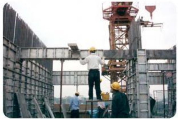
安装顶板、梁底板 The Assembling of the Slab and Beam Soffit
