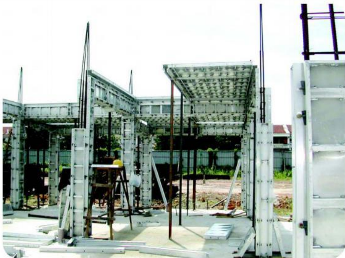
柱、梁、顶板 Column, Beam and Slab Panels in the Project
