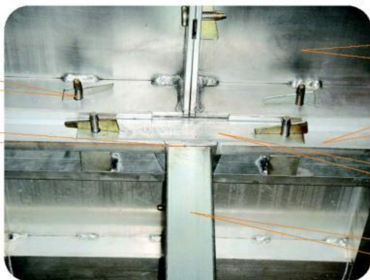
晚拆头连接形式 The Connection Way of Panel Prop Head
