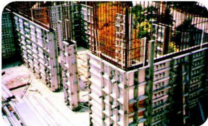
按顺序安装竖向模板 The Assembling of Vertical Panels in Order
