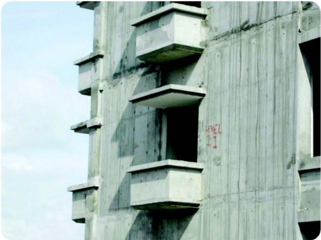
拆除模板后的效果 The Effect after the Formwork Dismantling
