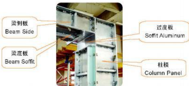
梁柱相交 Beam and Column
