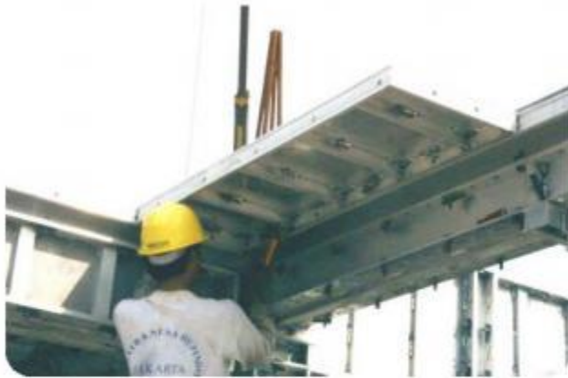
安装顶板、梁底板 The Assembling of the Slab and Beam Soffit
