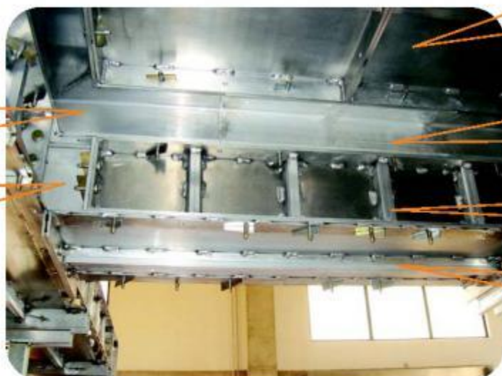
梁侧板、顶板转换连接 The Connection between Beam Side and Slab Panel
