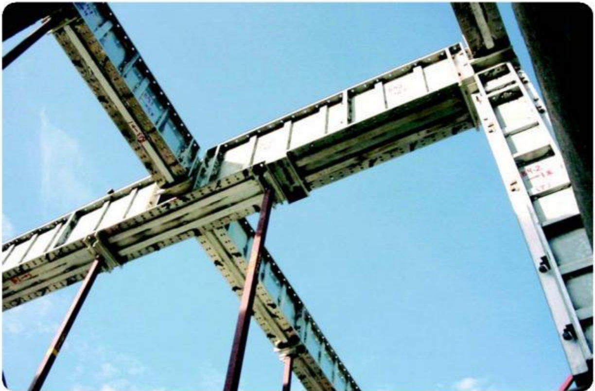
梁、柱模板的安装 The Installation of the Beam and Column Panels
