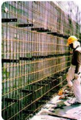
安装完单侧墙模板 The Assembled Single-sided Wall Panels
