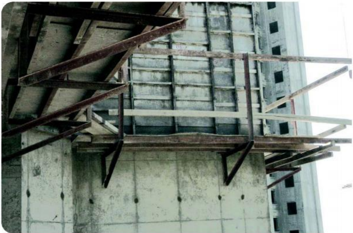
外側模板可用懸臂架或外挂架 The Both Light and Top Cantilever Bracket Could Be Used at the Outer Wall
