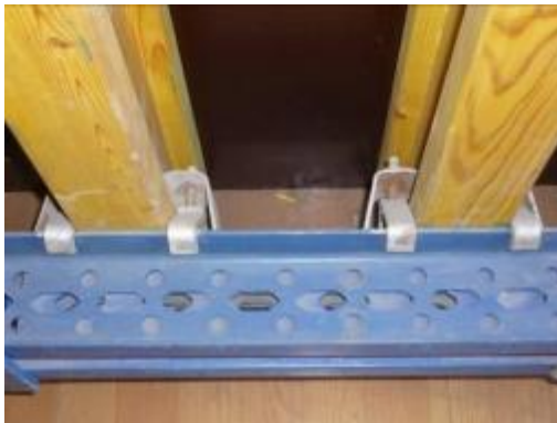
木梁与槽钢背楞采用专用扣件连接 The connection between wood H beam and channel waler adopts special connector.
