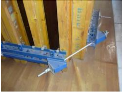
转角处，两模板间采用阳角对拉器连接固定 Angle Tie Bracket is adopted to connect the formwork when there is a corner.
