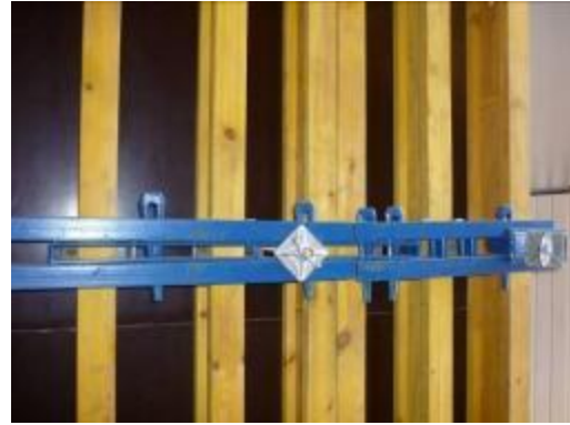
模板间采用芯带连接，并用钢销固定 The connecting plate are used to connect panels, and with pins to fasten the connection.
