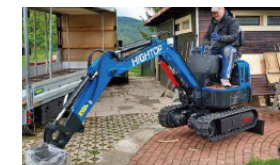
Our excavator in Spain.
