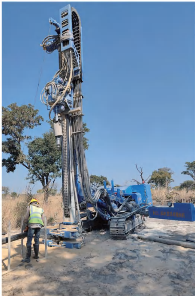
注浆引孔施工 Grouting pilot hole construction
