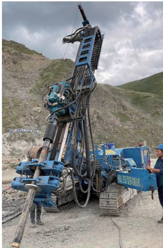
旋喷引孔施工 Grouting pilot hole construction
