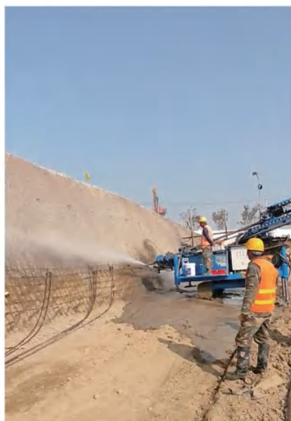
边坡锚索 Slope anchor cable
