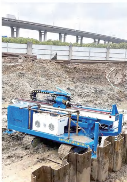
基坑旋喷锚索 Foundation jet-grouting cable
