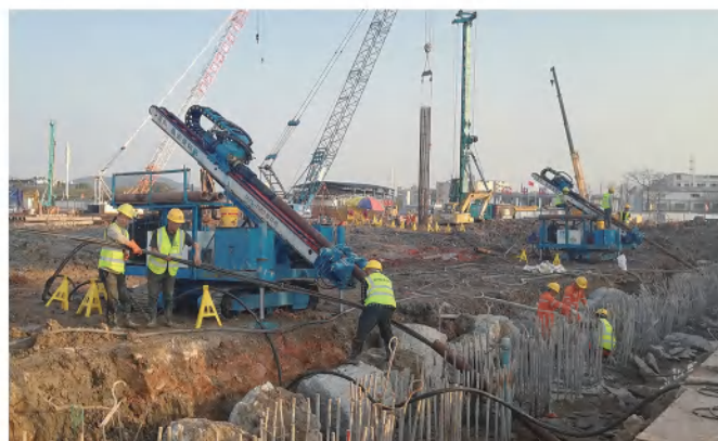
基坑斜锚索施工 Inclined anchor cables in foundation pits
