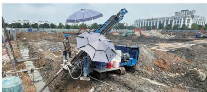
基坑锚索 Grouting pilot hole construction
