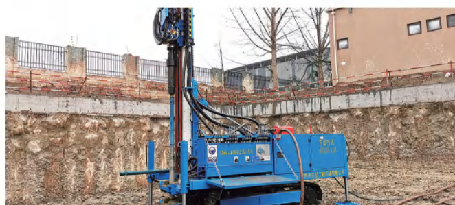
抗浮锚杆 Anti-floating anchor rod
