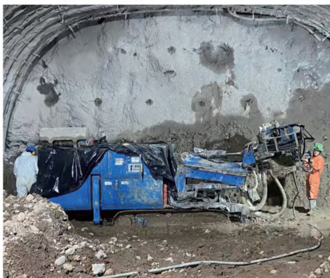
隧道超前注浆 Tunnel Advance Grouting
