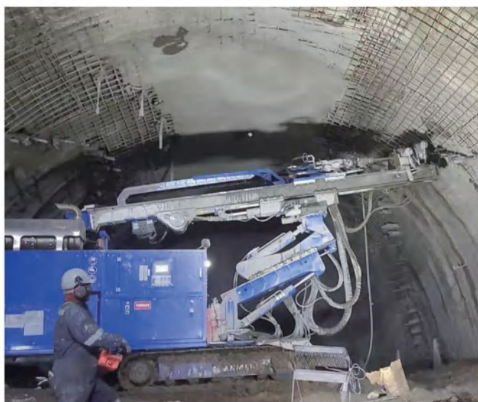
隧道超前注浆 Tunnel Advance Grouting
