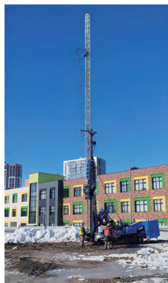
旋喷加固 Jet grouting reinforcement
