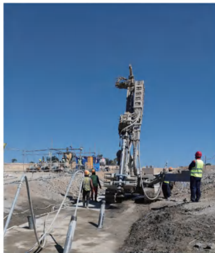
灌注引孔 Cast-in-place pile pilot hole
