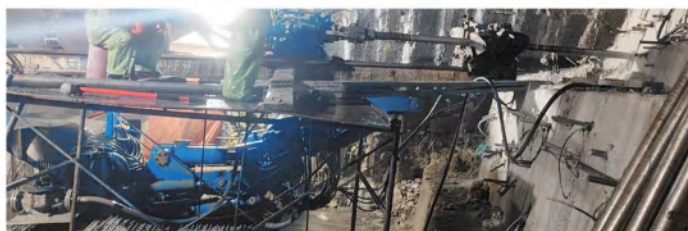
隧道注浆 Tunnel grouting
