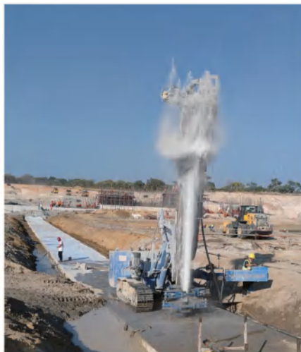
灌注引孔 Cast-in-place pile pilot hole
