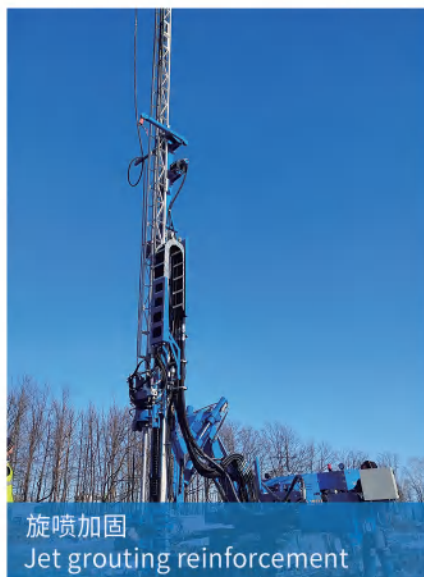
注浆引孔 Grouting pilot hole
