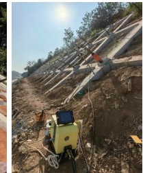
On site equipment installation
