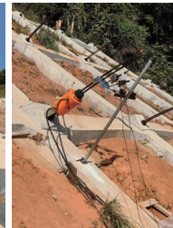
Installation of displacement sensors
