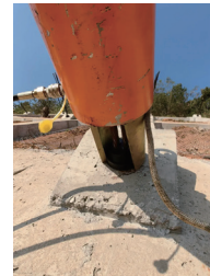
Installation of support bench and jack
