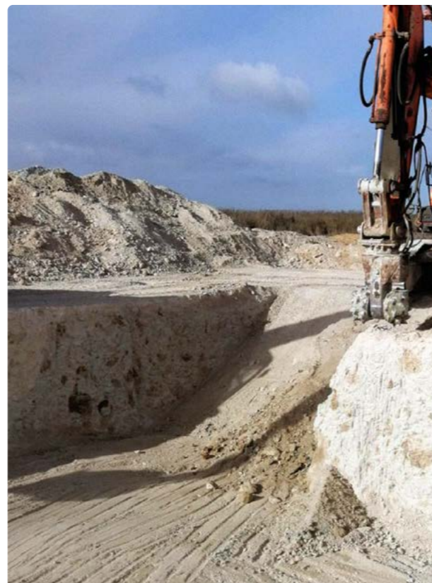
Images above: A KRD 120 MIX producing consolidated soil structures using the MSM process
