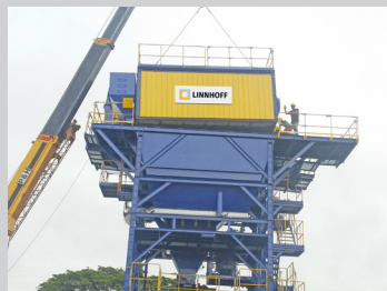
Baghouse filter module
