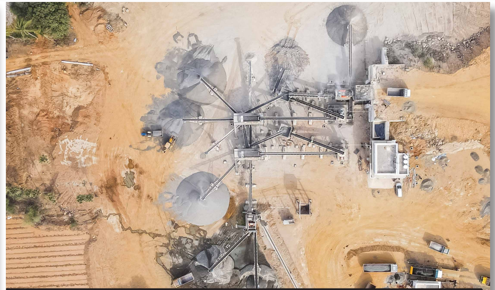
350 TPH - 3 STAGE C&S PLANT WITH WASHING SYSTEM
