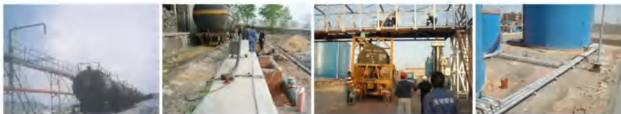
火车装油平台 Railway bitumen loading platform
