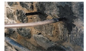
Cement slurry injection at controlled pressure
