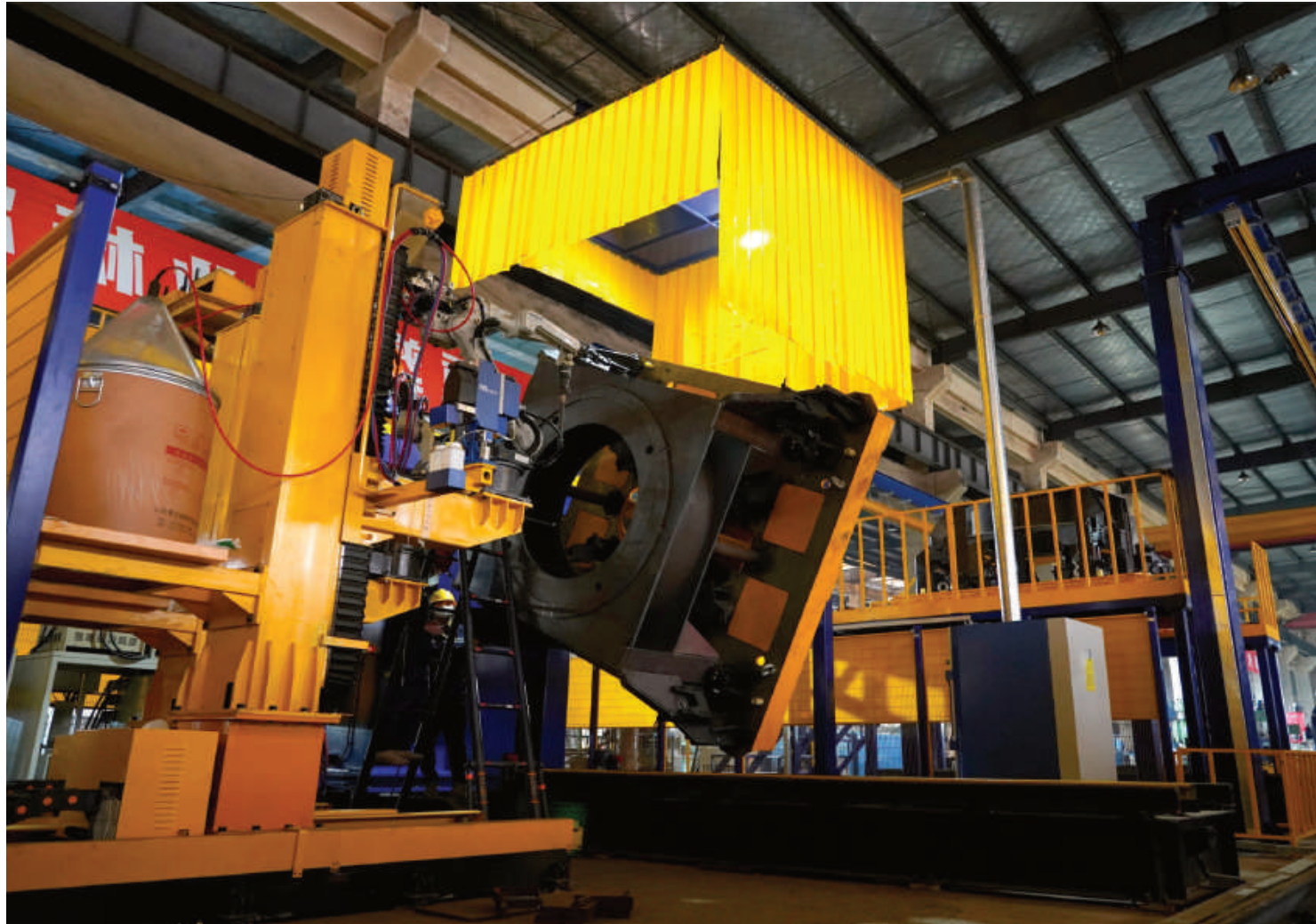
Upper and Lower Slewing Assembly Welding Automation Line
