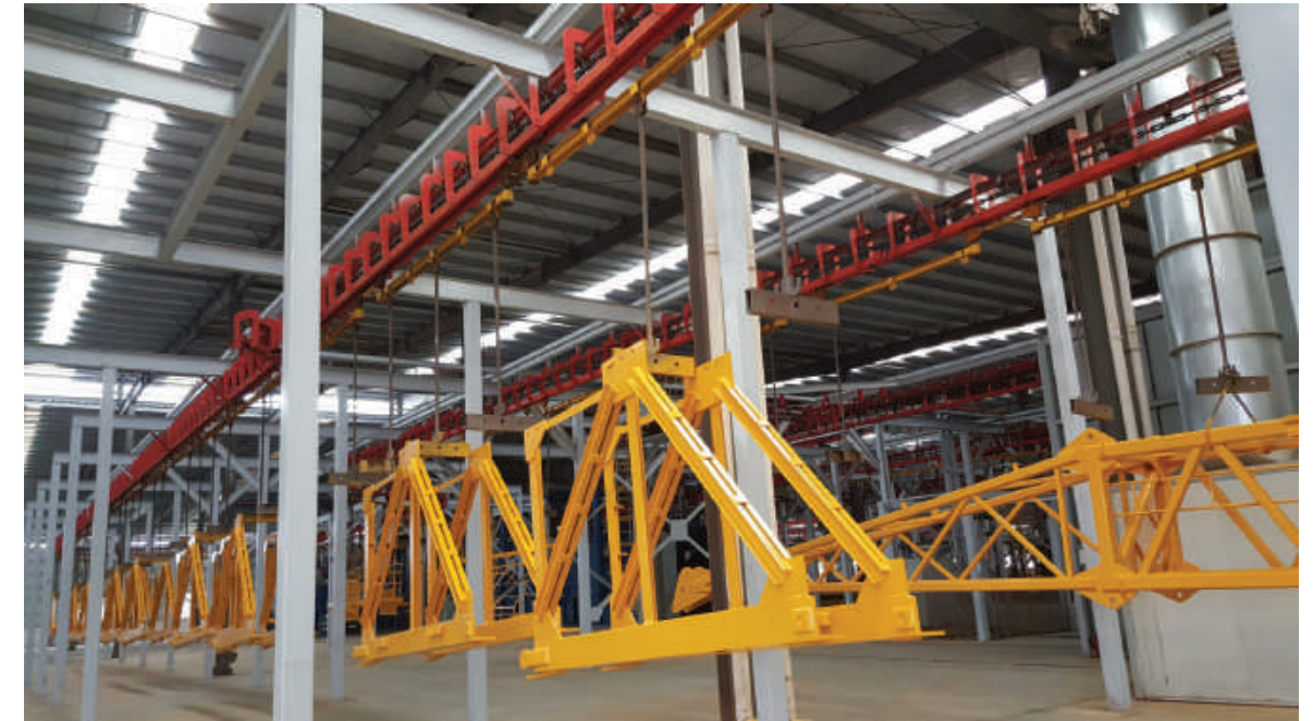
Steel Structure Shot Blasting & Coating Post-processing Center
