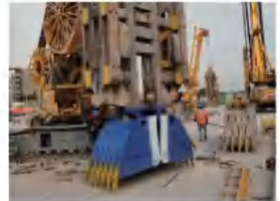
佛山西江水利工程 Foshan Xijiang River Hydraulic Engineering Project
