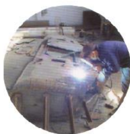
焊接外壳 Welding Shell
