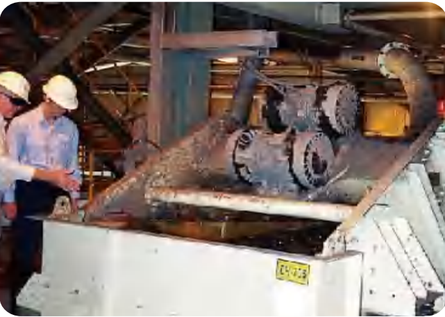
[ 设备安装调试 ] Equipment installation
