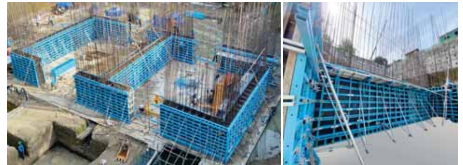
► Project in the Philippines
