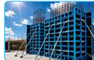
5 Wall Formwork
