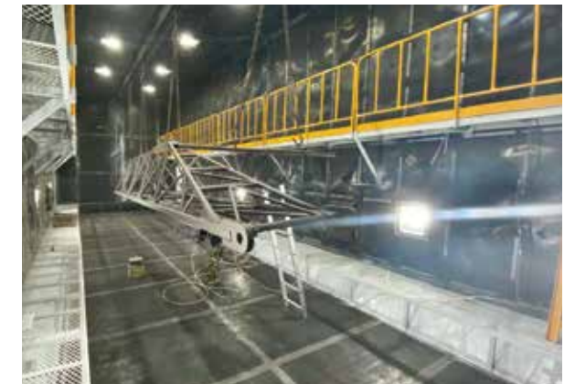
抛丸打砂 Shot blasting
