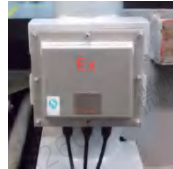
防爆接线盒现场 Explosion-proof junction box
