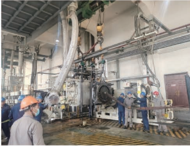
换网器拆除保养 Dismantling and Maintenance of Screen Changer
