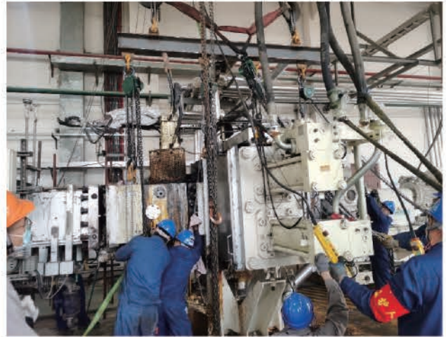
开车阀拆除保养 Dismantling and Maintenance of Start-up Valve
