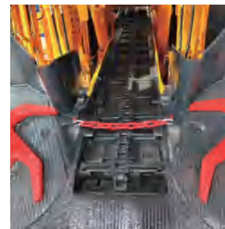
掘进机 Tunnel Boring Machine
