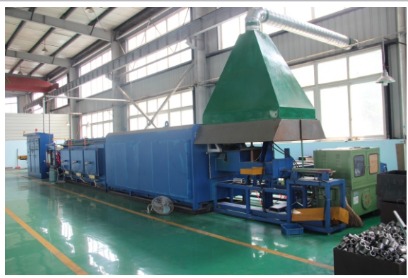
烧结炉 Welding furnace
