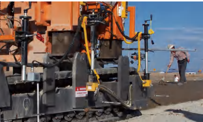
6.Auto leveling and tracing systems ensures paving surface flatness and road straightness.
