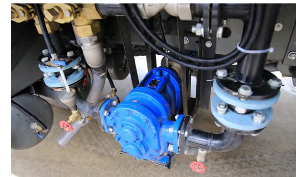
3. The asphalt pump is connected to the engine for heat preservation, and the work efficiency is higher.
