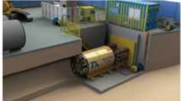
安装顶管机主机 Installation, connection and debugging of pipe jacking machine
