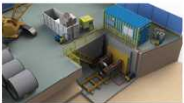
安装始发井内组件 Install auxiliary equipment in starting shaft
