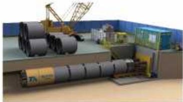
长距离顶进，安放中继间 Install inter jack station
