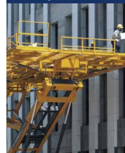
Office building wall construction
