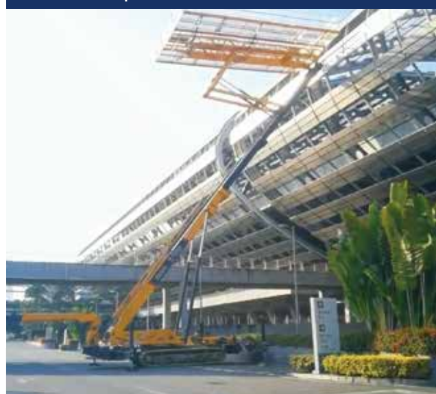
Canton Fair Complex renovation and maintenance
