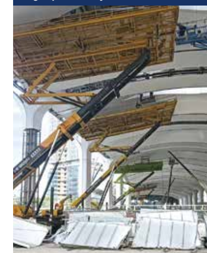
High-speed railway station construction
