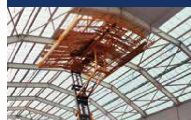
Traditional construction methods
