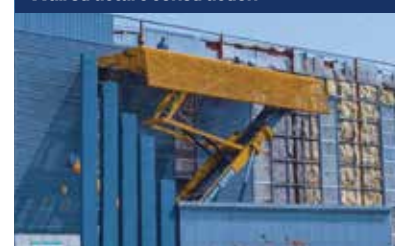
Wall structure construction
