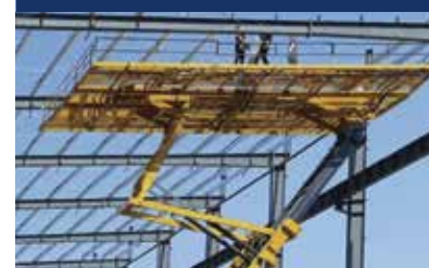
Roof structure installation
