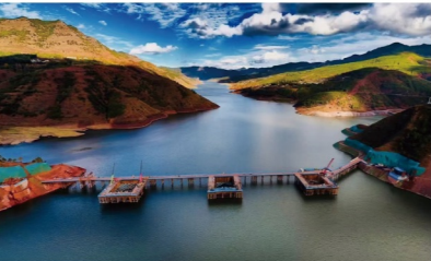
Maojiacun Reservoir Major Bridge Cofferdam
