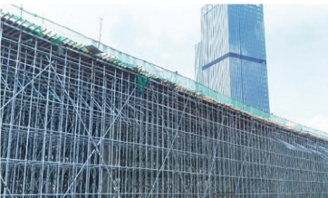
Hangzhou Xiaoshan Airport Expressway
