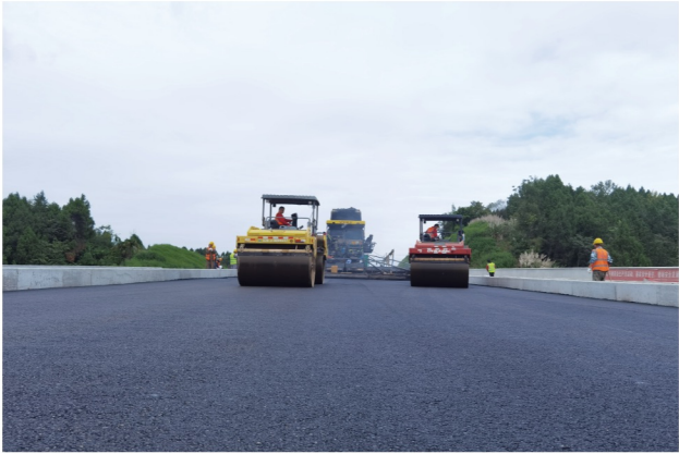
CCCC Second Harbor Company Co., Ltd. - Jintang-Jianyang-Gaoxin Expressway
