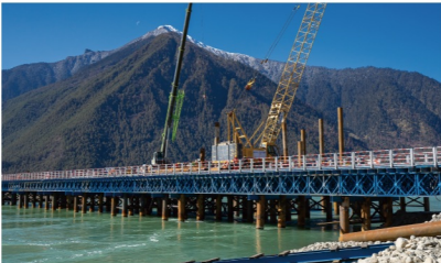
Yarlung Tsangpo River Major Bridge Project in Milin County, Tibet
