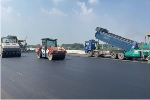
China Construction Sixth Engineering Division, China Railway No.10 Engineering Group Co., Ltd - Qingdao 204 Daogu River Bridge
