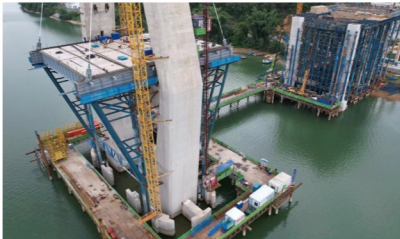
Shanglin-Hengzhou Expressway Xijin Yujiang Bridge Side Beam Steel Support
