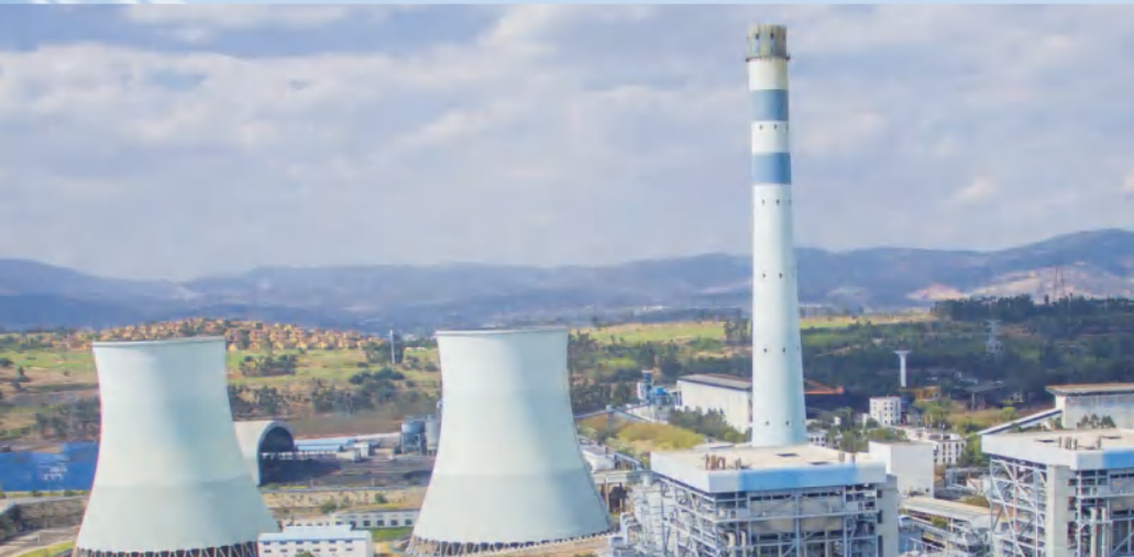
燃煤发电 Coal-Fired Power Generation
