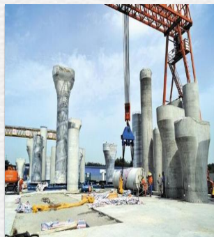
路桥工程领域 Road&Bridge Engineering
