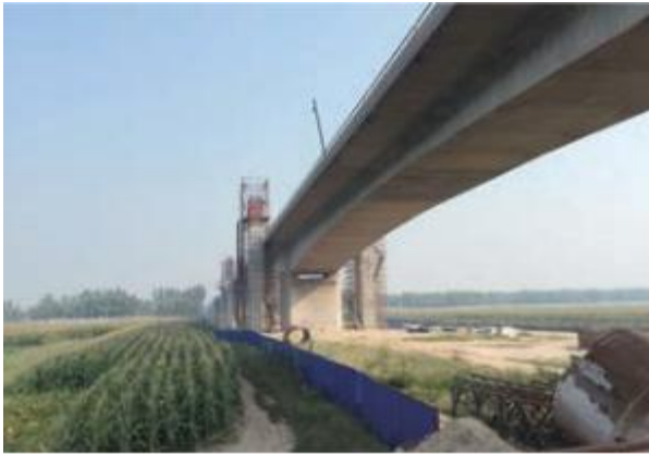
Reconstruction Project of Dongming Yellow River Bridge
