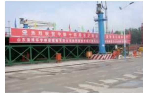
Beijing-Shanghai High-Speed Railway
