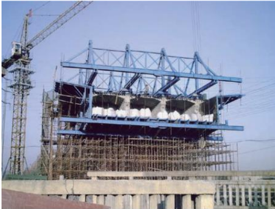
Construction site of Form Traveler for China Railway Tenth Group
