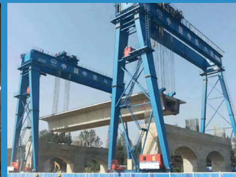
500t concrete beam lift
