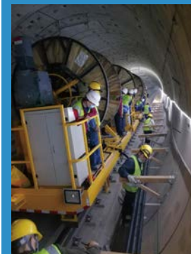
Automatic Cable Laying Vehicle
