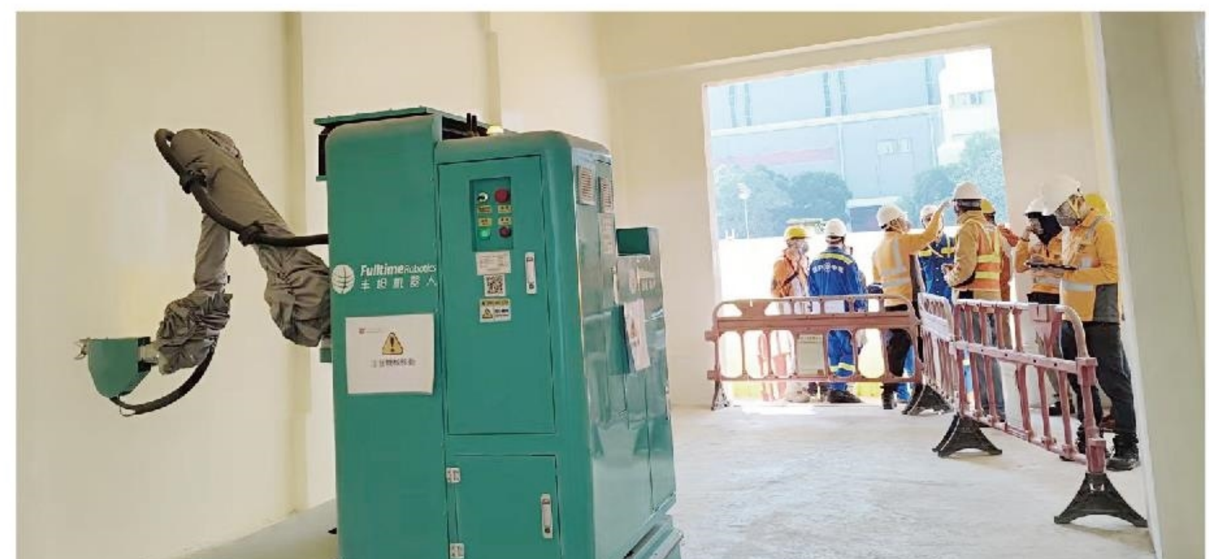
CPPS FS Tank A&A work, Hong Kong
