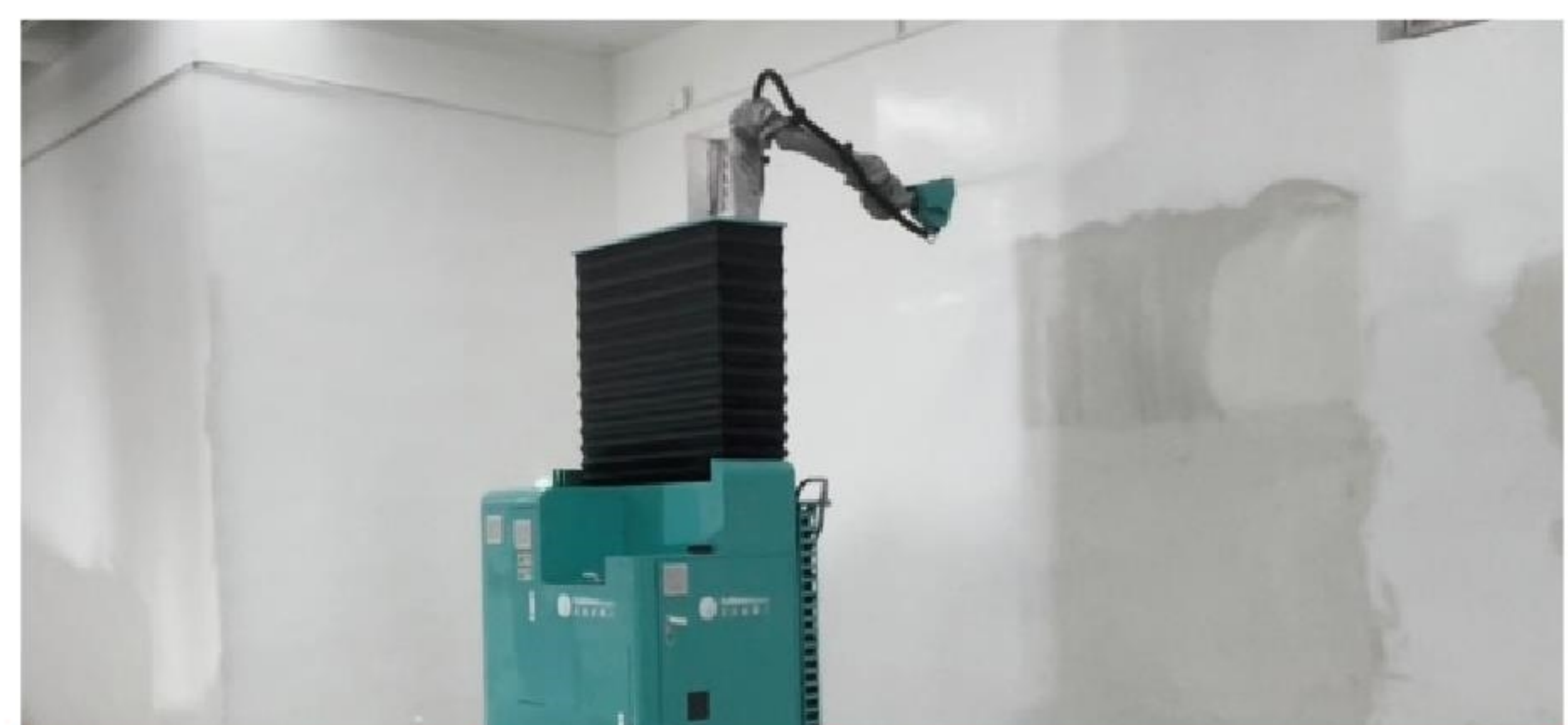
Sanxiang Kowloon Freight Centre Warehouse, Hong Kong
