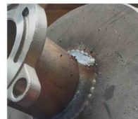
角焊缝气保焊
