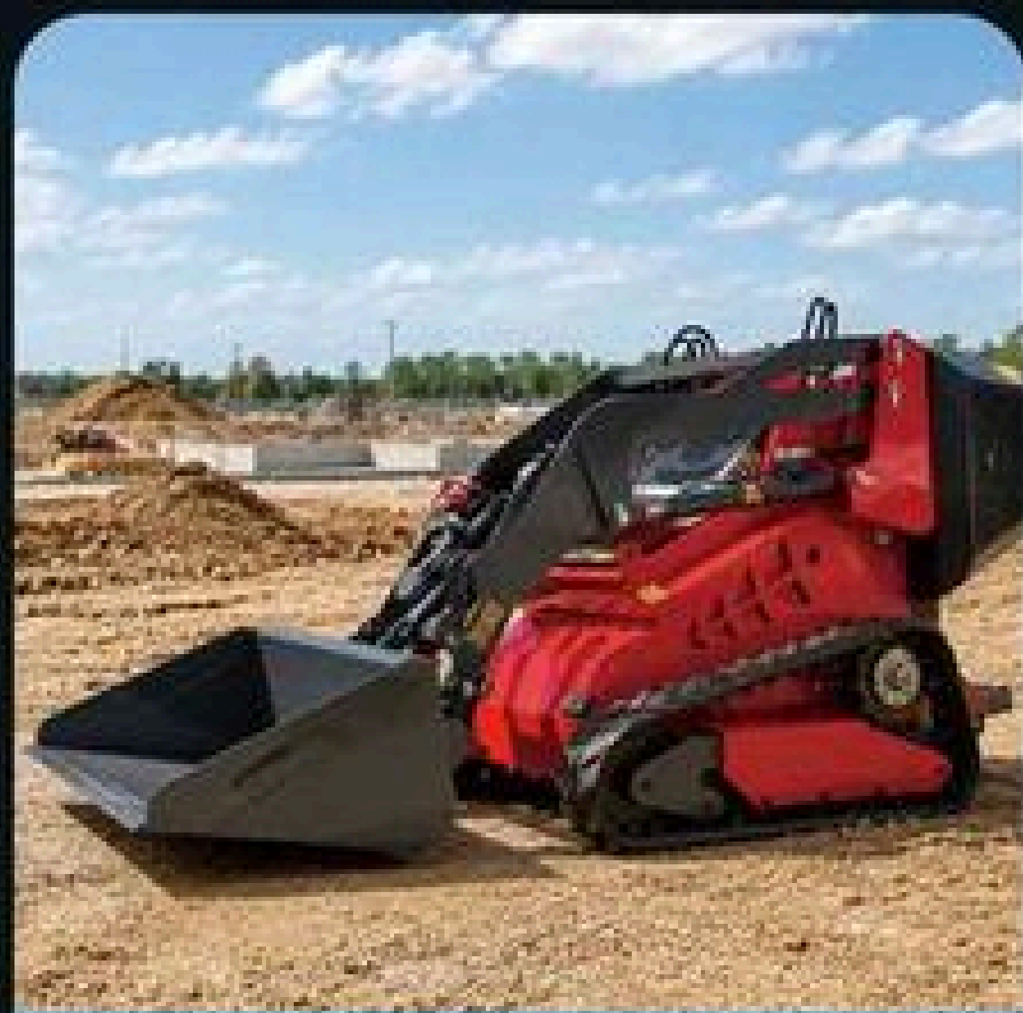
工地/Construction site
