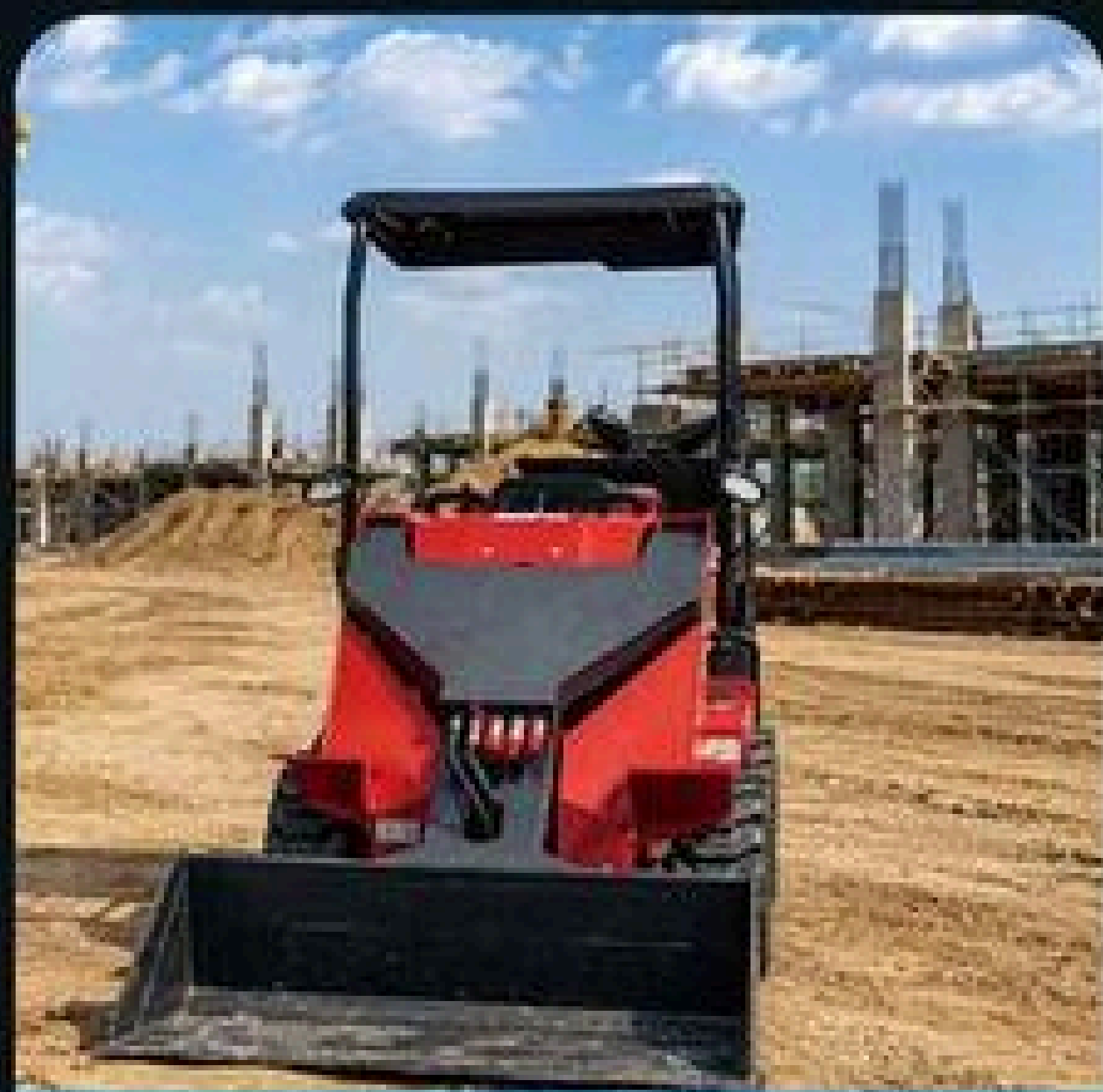
工地/Construction site
