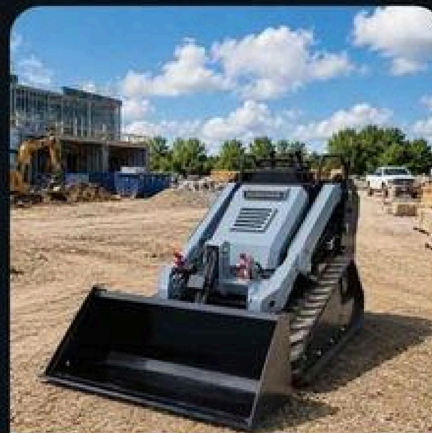
工地/Construction site
