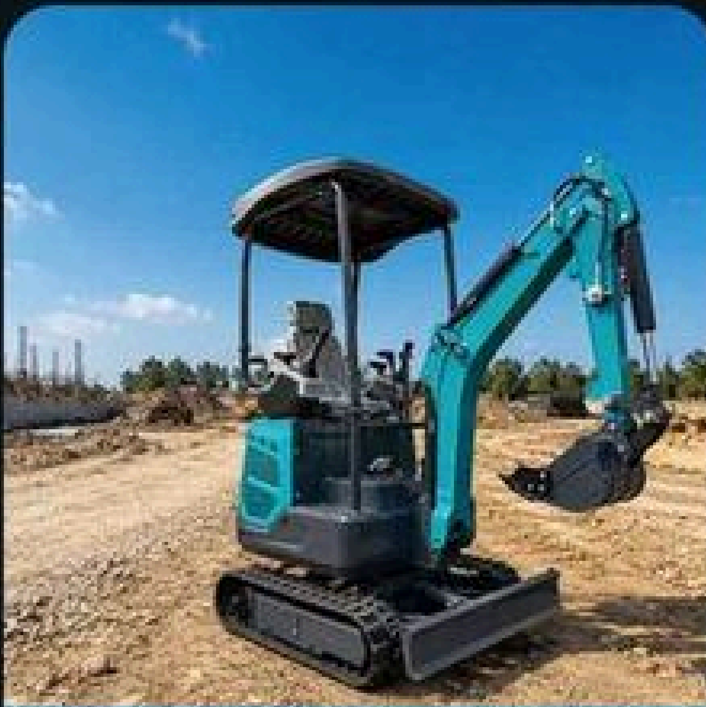
工地/Construction site
