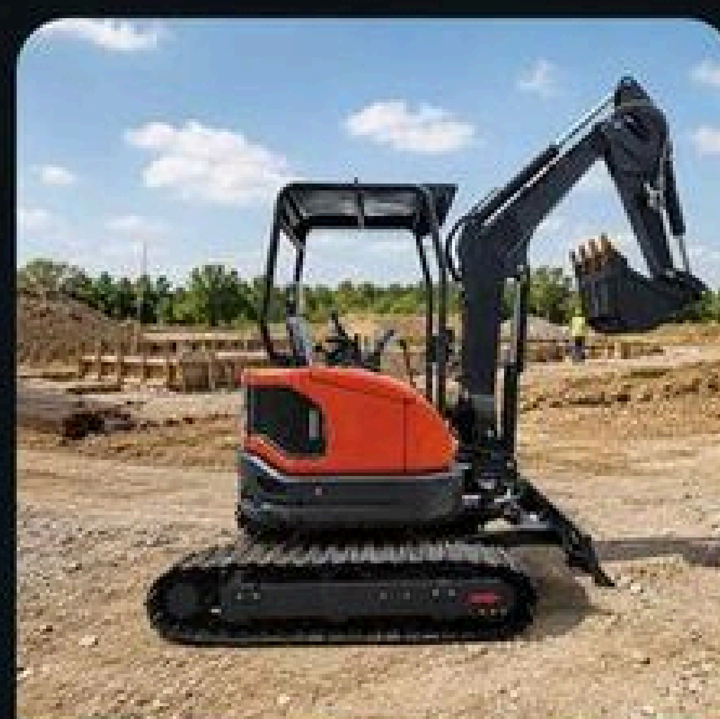
工地/Construction site
