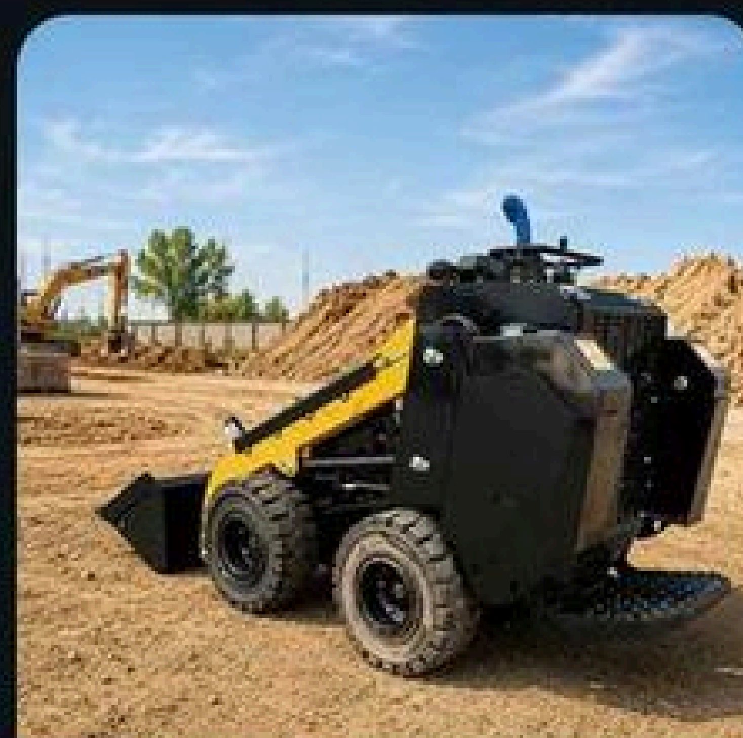
工地/Construction site
