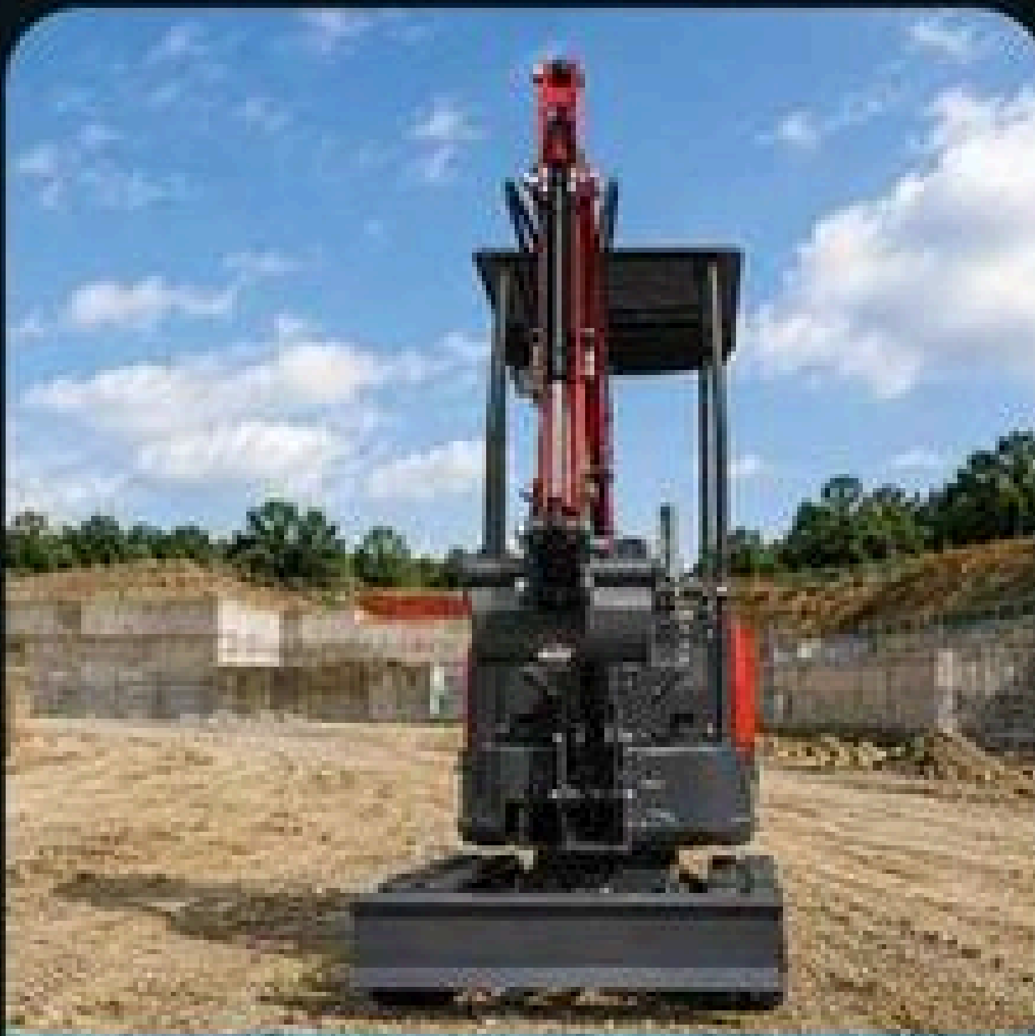
工地/Construction site
