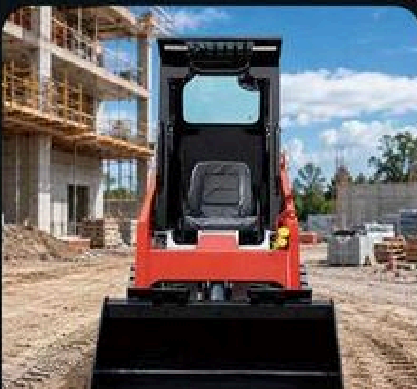
工地/Construction site
