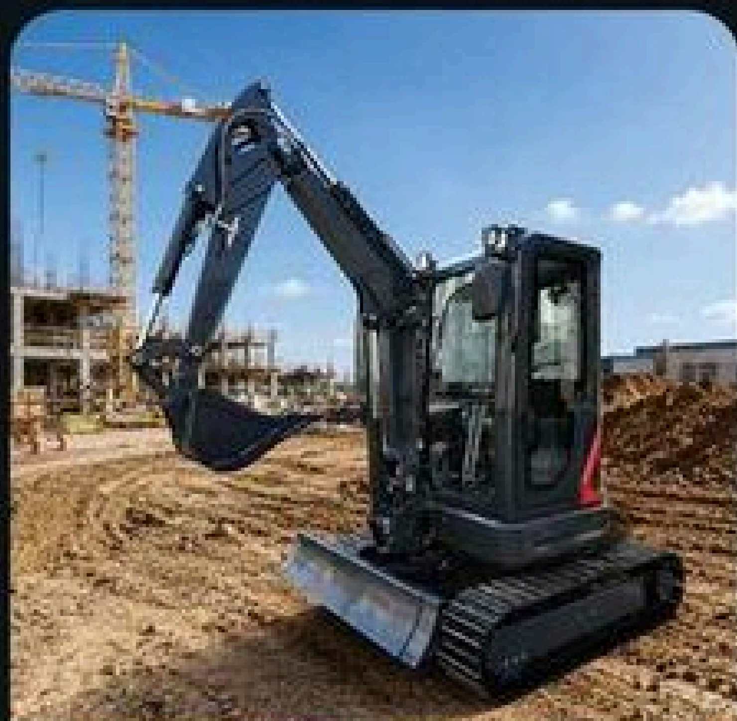
工地/Construction site
