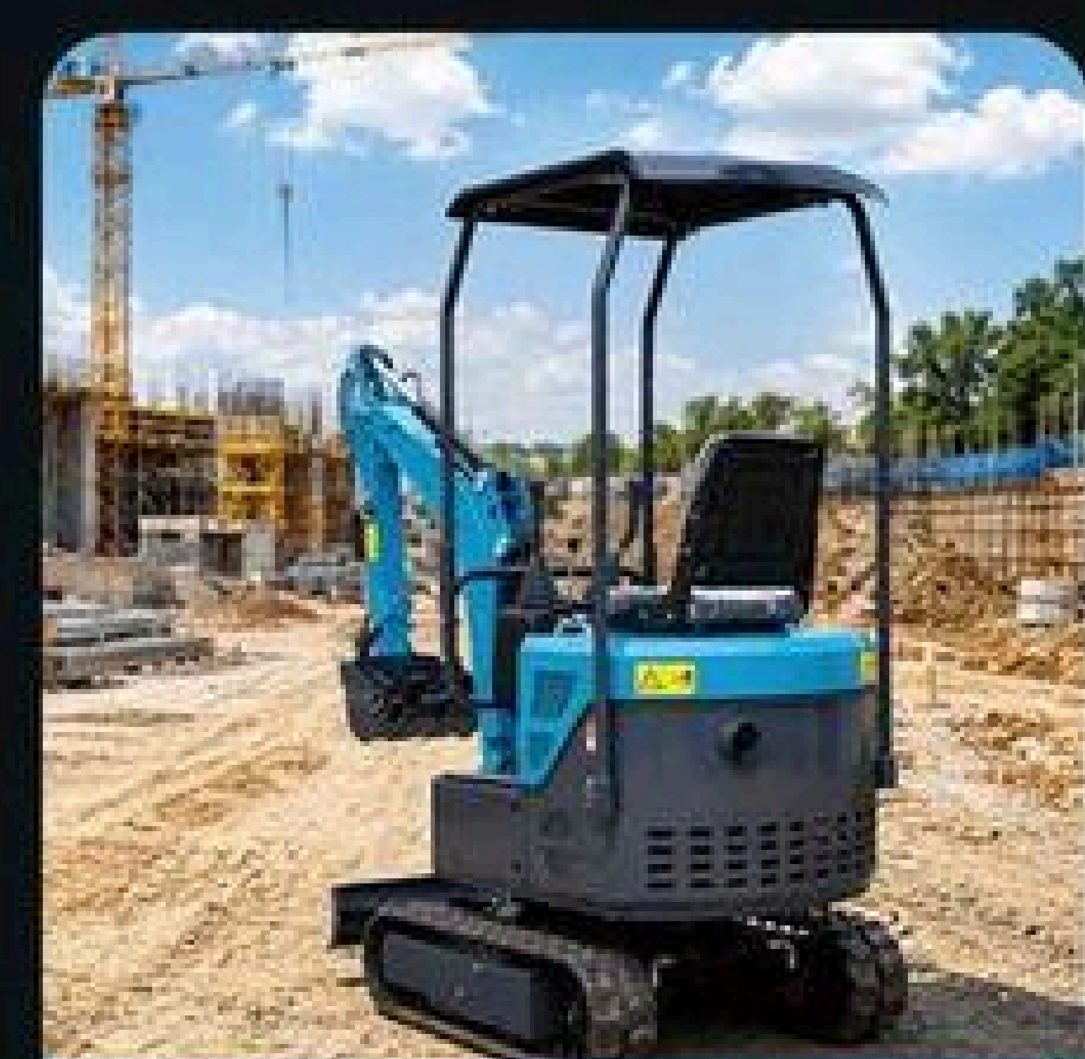
工地/Construction site
